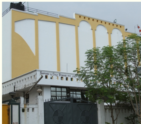
REFRIGERATED WAREHOUSE (Navi Mumbai)
